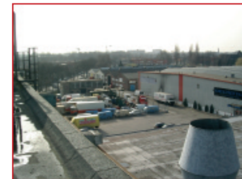
The Volt/Phoenix complex – Tilburg
