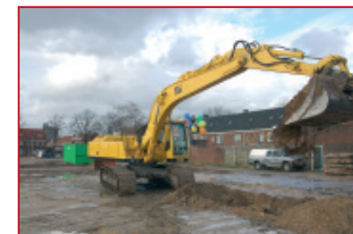
Site preparation – Tilburg
