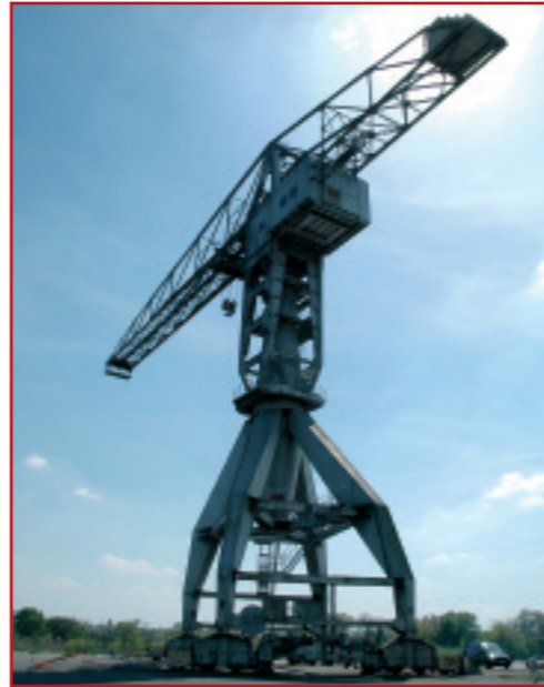
The Grey Titan Crane on the former Nantes Shipyards site – Île de Nantes
