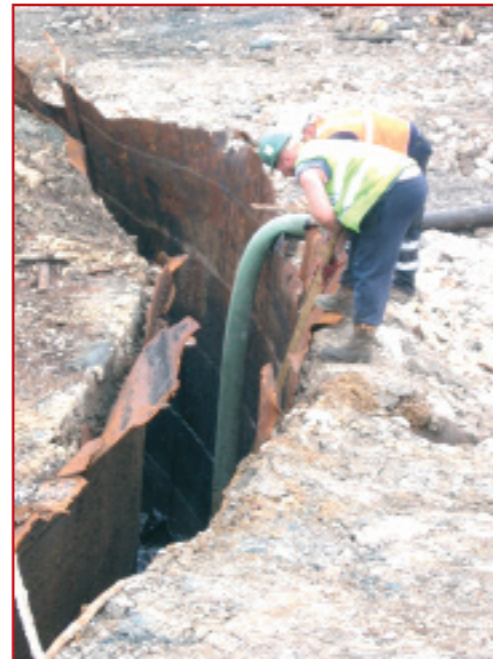
Removing contaminated groundwater from dismantled gas-holders – Medway
